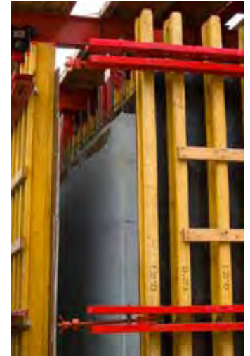
Forms, separated from the core, are ready to move up.
