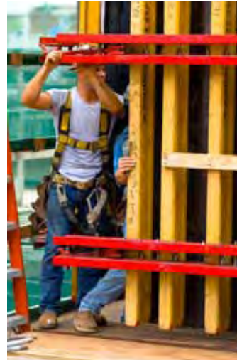
Core crew breaks and moves exterior forms.
