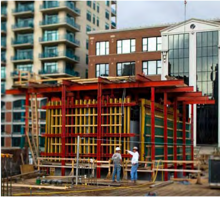
The Self Rising Core System frees up crane time on the job, increases efficiency and enhances safety.
