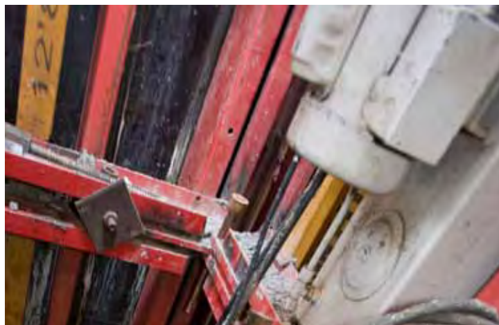
Hydraulic cylinder units allow movement to the next pour level without the use of your tower crane.
