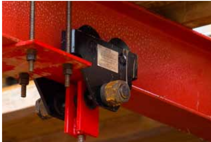
Trolleys, supported by grid beams, are attached to exterior forms.
